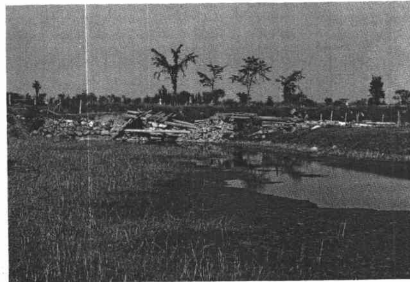
Farm Bridge Across Rivière Delisle was Destroyed by Fast Flowing Flood Waters.
